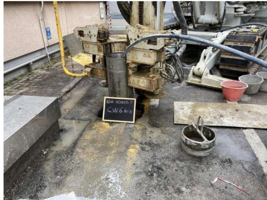
Posa piezometro 3 pollici e dreno siliceo / Installation of 3" pipe and drain
