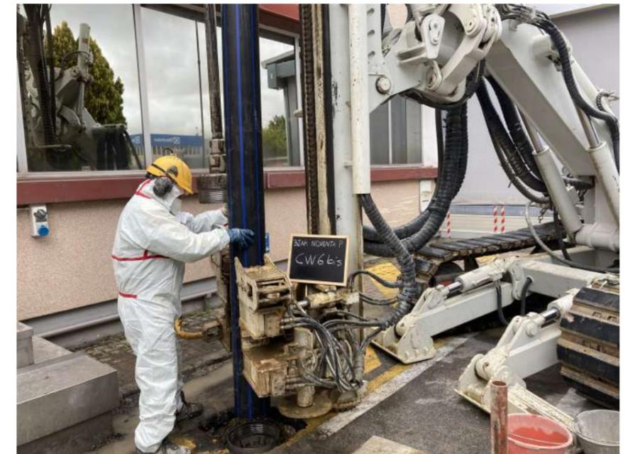
Cementazione del tubo cieco HDPE / Grouting of the HPDE pipe
